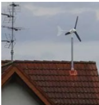
Roof-mounted wind turbine
