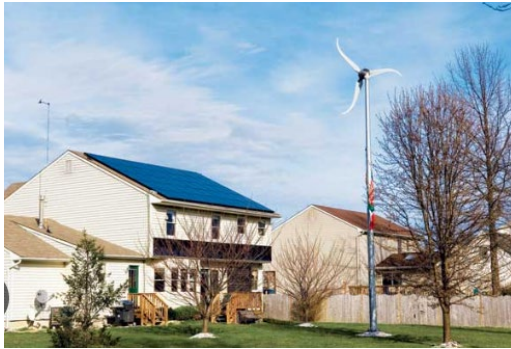
Roof-mounted solar and ground-mounted wind
