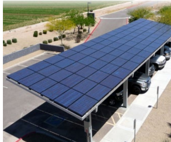
Carport roof-mounted solar
